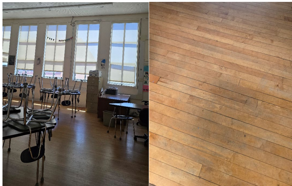
Pacific Grove Middle School Classroom Flooring
