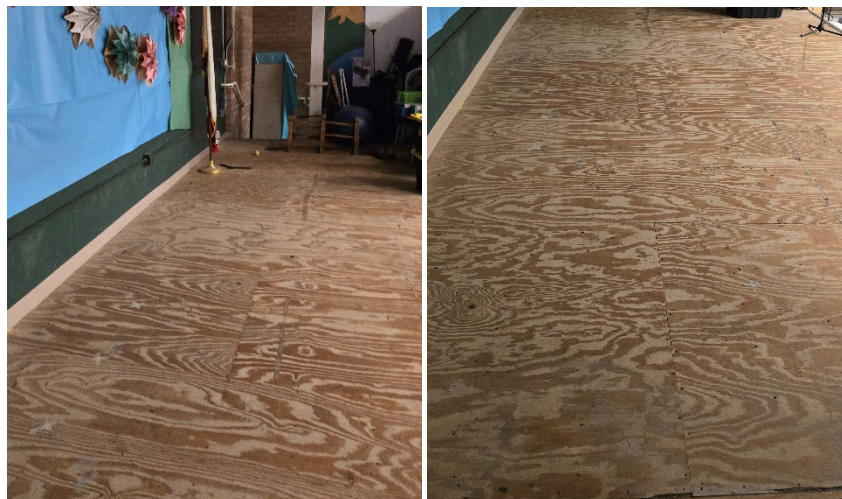
Forest Grove Elementary School MPR Stage Floor
