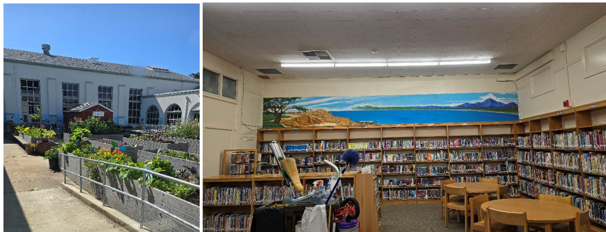
Robert H. Down Elementary School Courtyard and Library
