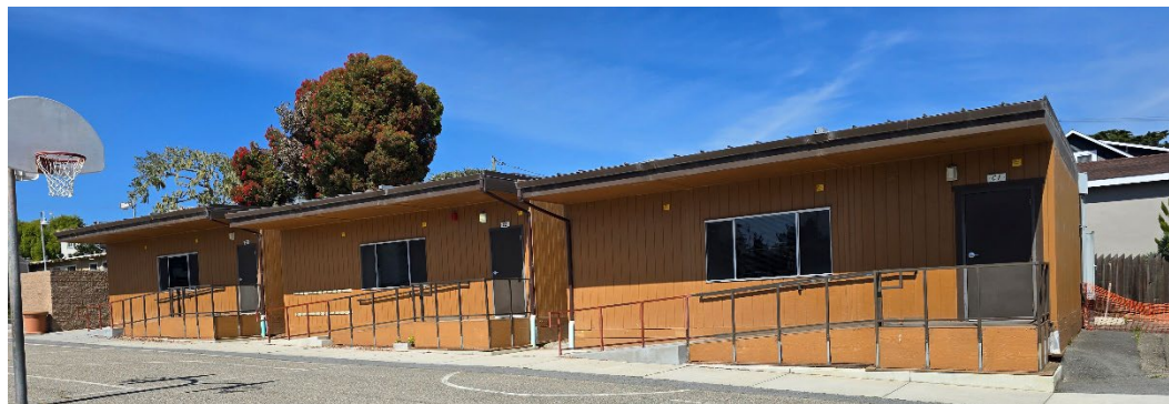
C-Wing Relocatable Classrooms
