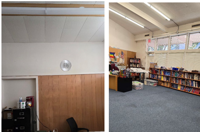
David Avenue School Classroom Finishes
