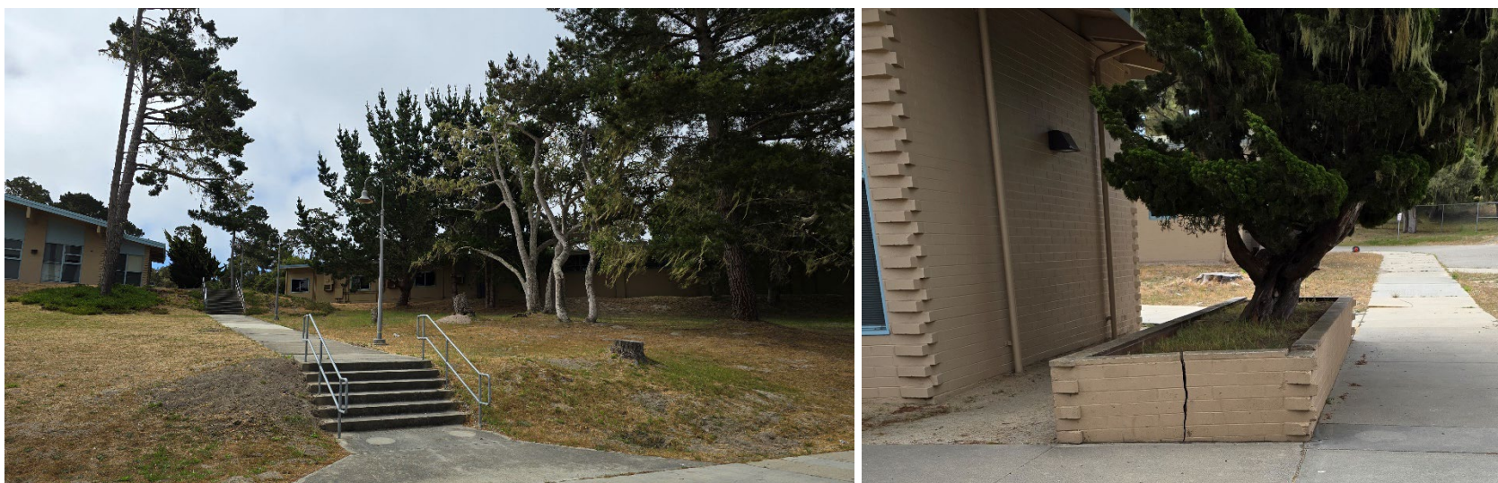
Pacific Grove High School Grounds Conditions
