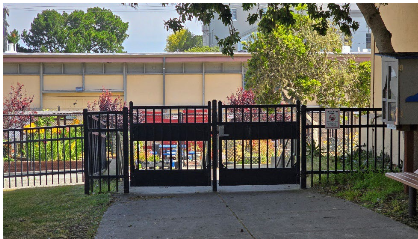
Pacific Grove Middle School 4 ft. Perimeter Fence and Gates
